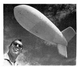
PROTOTYPE BALLOON was used to support air blast pressure gages during HE detonations at Coyote Test Field.
